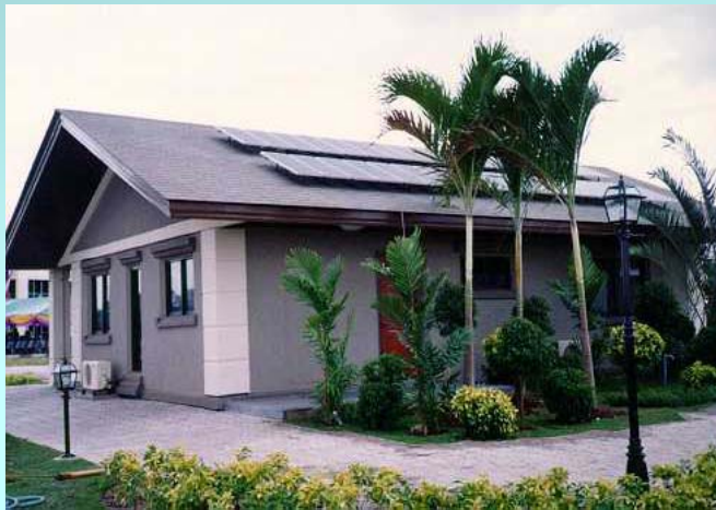
Vanadium Battery Powered Solar House in Thailand (1993)
