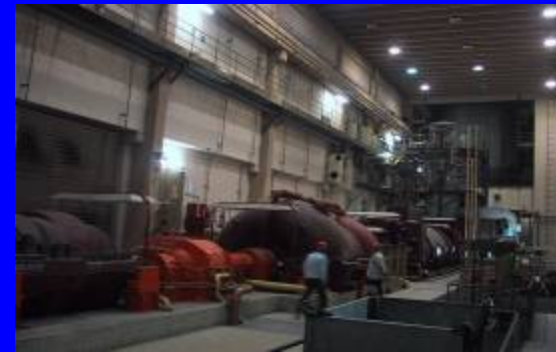
Huntorf, Germany, 290 MW
