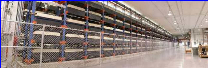
40 MW in Fairbanks, Alaska
