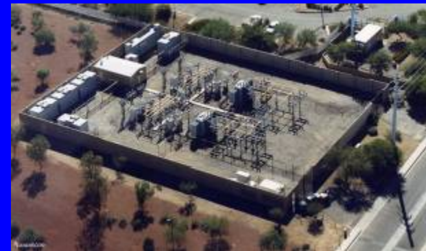
10 MW - 30 sec at Microchip Plant
