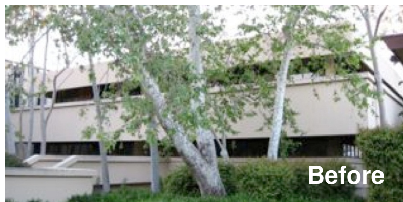
Jorgensen Laboratory Building
